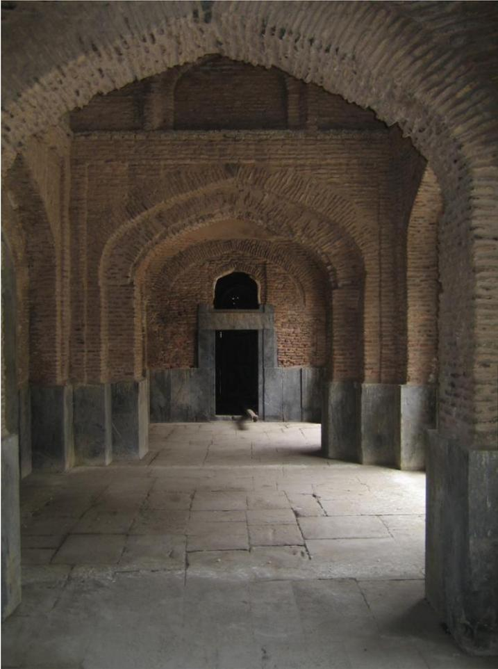
**Fig. 86: Mullah Shah Mosque: Interior view at colonnade with brick core revealed**
