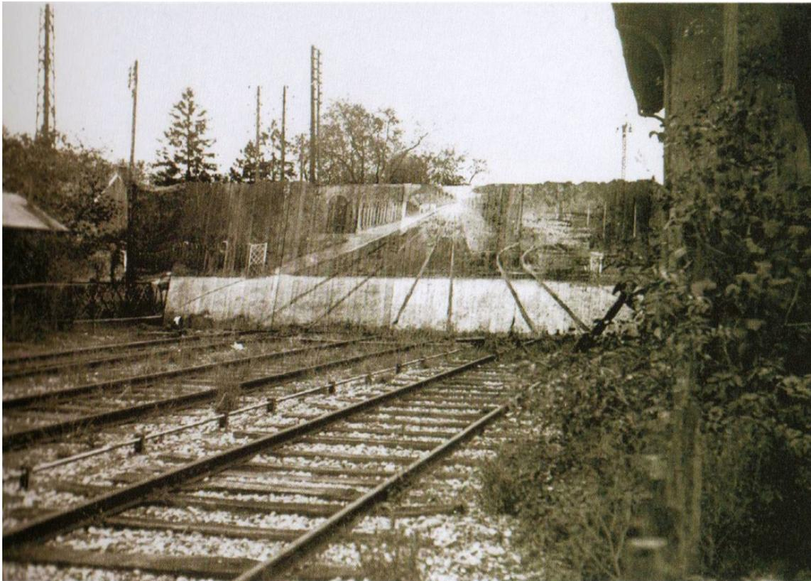
Trompe l'oeil railway lines at Pont-a-Mousson Station, 1915 used to disguise presence of munitions trains.
