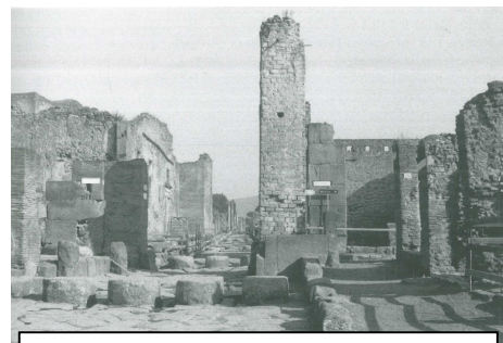
Abb.17 Wasserturm in Via Stabiana
