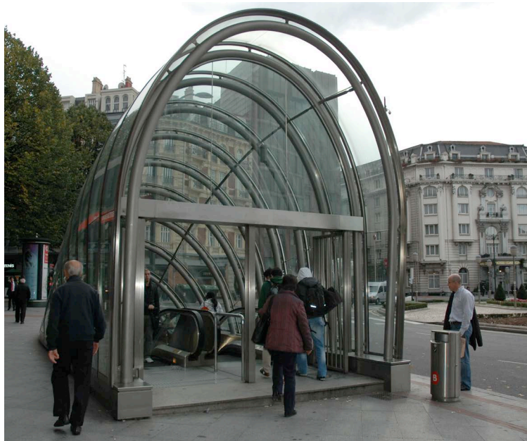
Abb. 5: Norman Foster & Partners, U-Bahn Abgang, Bilbao, 2005
