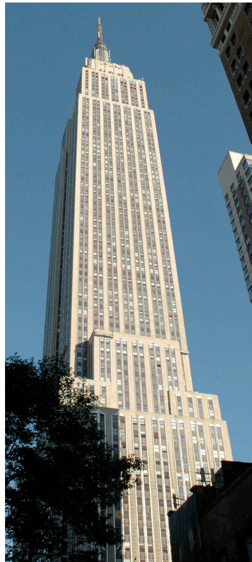
Abb. 148: Shreve, Lamb & Harmon, Empire State Building, New York City, 1931
