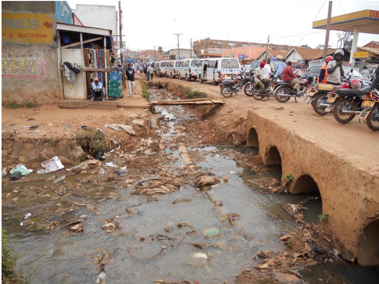
Picture 3: Drainage System in Kawempe, a GKMA Slum Area, 2010
