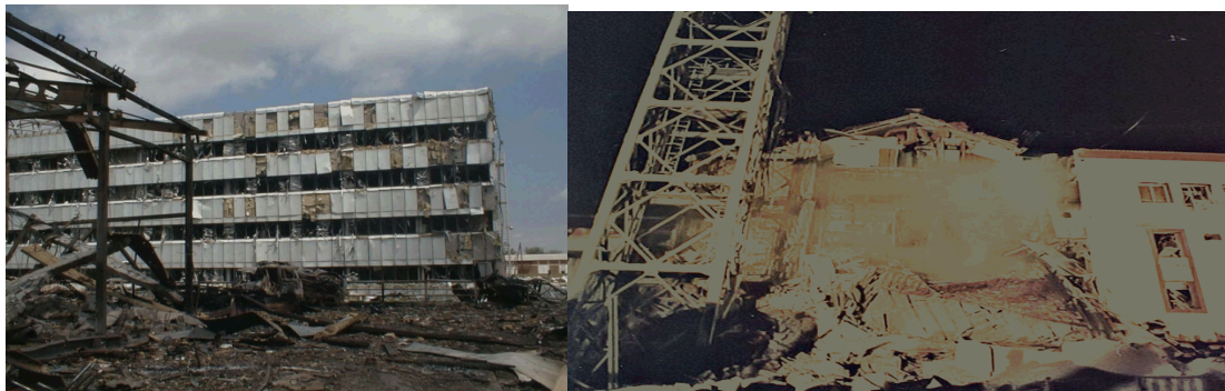
Figure 5: TV studios of the Radio-Television Serbia in Novi Sad and Belgrade destroyed by NATO in 1999
