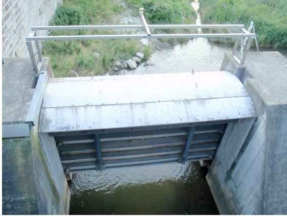
Pic. 11 A weir-shutter in opened position at the flood-control reservoirs.
