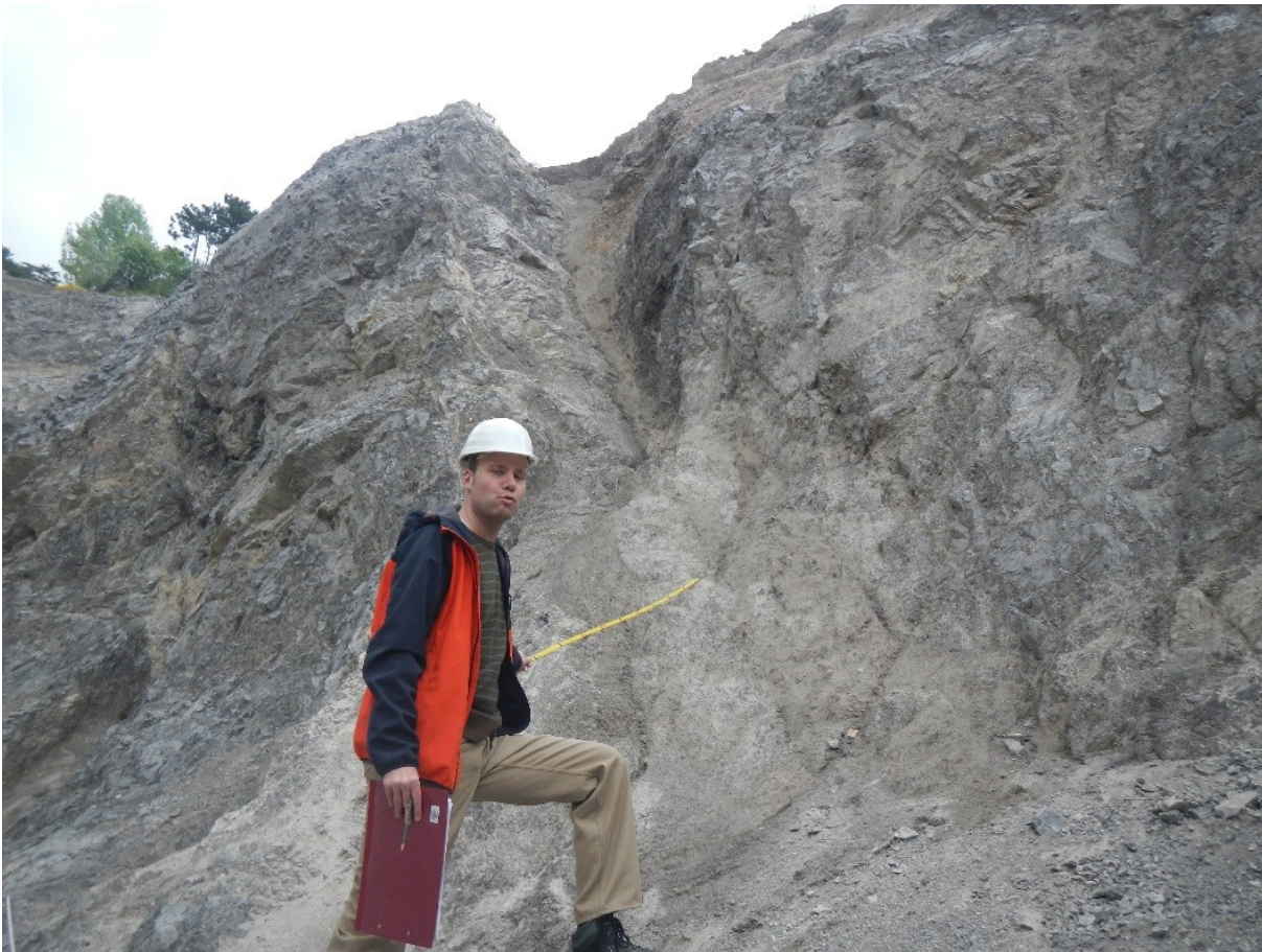
Figure 10: uncemented fault rocks often formed cones of washed out fault rock at their base showing a strong cohesion during dry weather.
