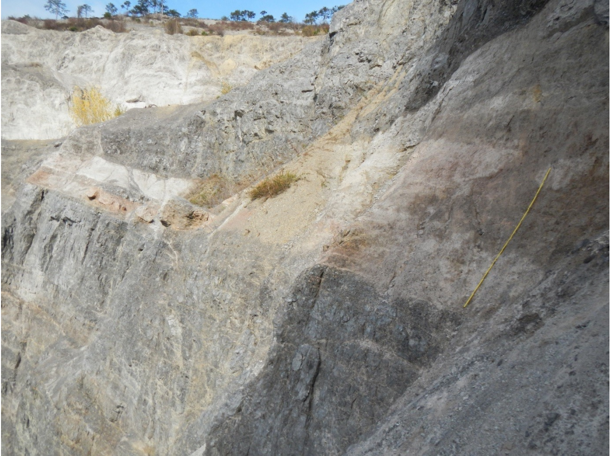
Figure 23: Bedding parallel fault rock with cataclasite of more than 2m apparent thickness in the eastern quarry wall (white next to measuring stick). View to N.
