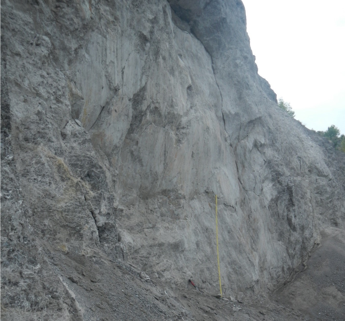
Figure 39: Apparently E-W striking fault system showing well developed fault rock, steep slickenlines and lunate fractures indicating downwards slip of the (missing) hanging wall. View towards ENE.
