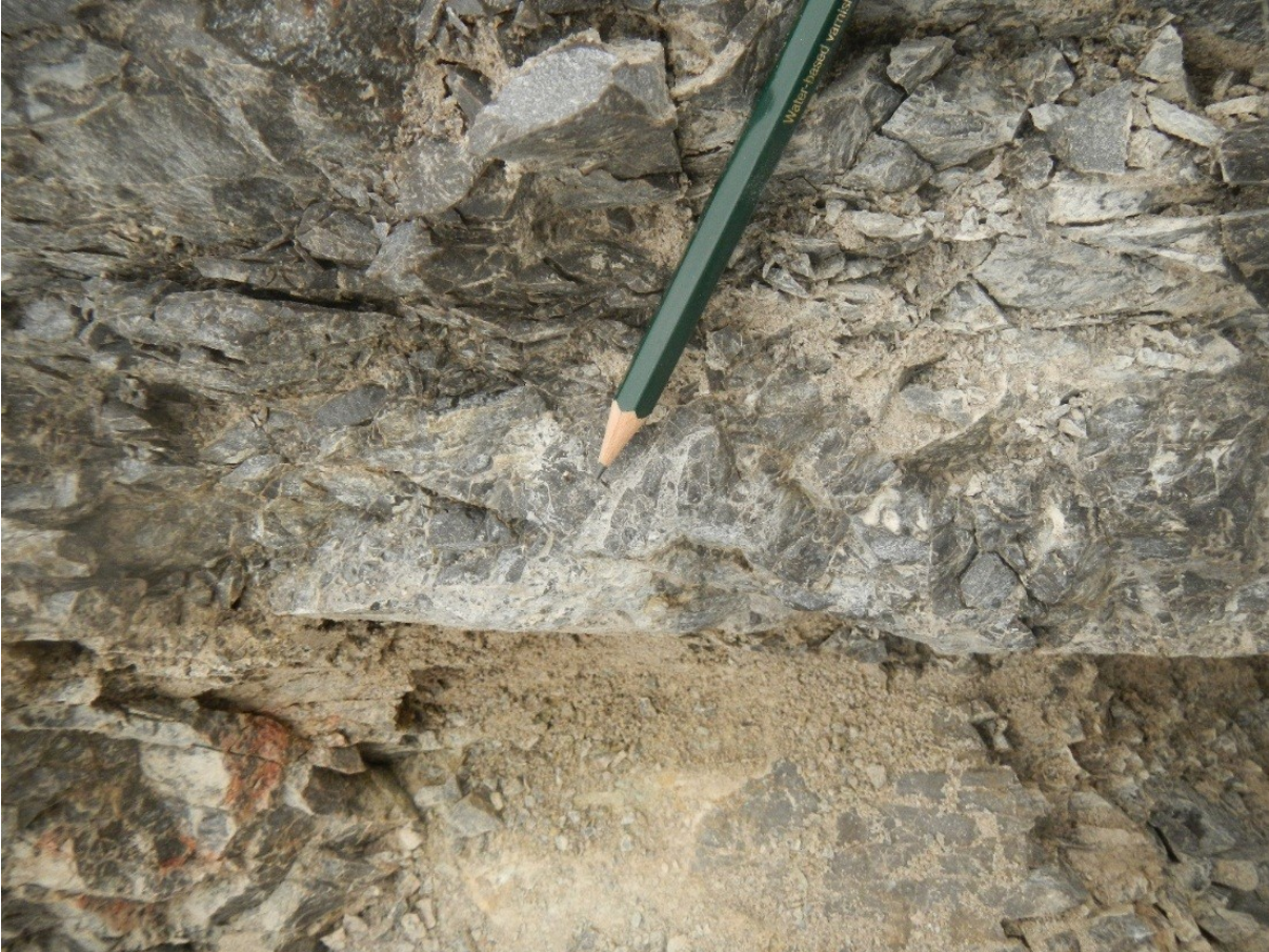
Figure 50: Looking down on the fault with samples 3 and 3.2 still in place. T-criteria indicate sinistral shear. The assumed tension gashes terminate in the protolith rock and are filled with the mature cataclasite forming the PSS. Tension gashes widen towards the fault and terminate at a distance of a few centimeters from the PSS. Note the presence of cemented and uncemented fault rock in the same fault pointing towards a reactivation postdating the cementation event. Note the thicker development of intermediate to mature cataclasite at the zone near the tension gashes (sample 3.2) and the dominance of the matrix to the right (sample 3) while bordering the same slickenside.
