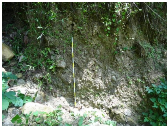
Figure 58: Fault scarp (tear-off edge) 2 m height
