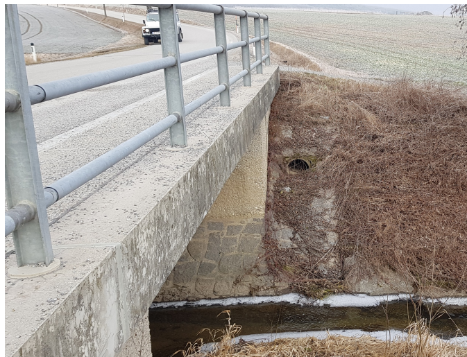
Figure 5.11: Entry point of a roadside ditch into the Funitz at a bridge close to the village of Oberhöflein (Foto: Humer 2018).
