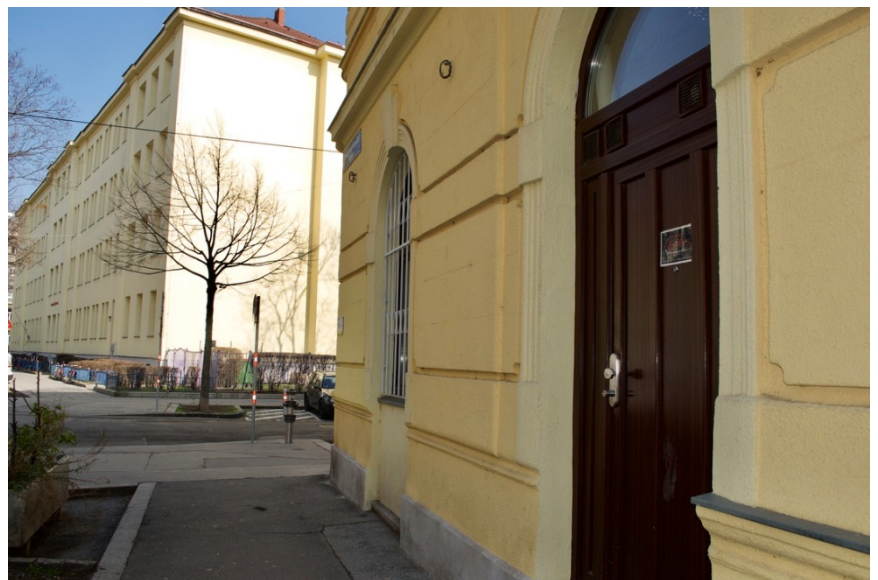
Figure 30. Laufhaus, Max-Winter-Platz, next to an elementary school (own representation, photo taken on 25 March 2021)
