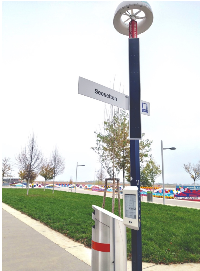
Figure VII: The smart stop equipped with IoT devices.
