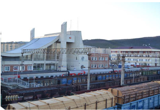
Figure 2. The railway station in Severobaikal'sk, symbolizing a ship's sail and designed by engineers from St. Petersburg. Photo by author.
