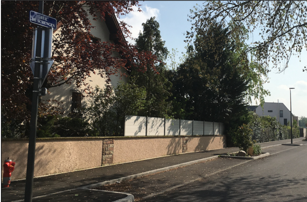
Figure 6. “Rue de Schengen” in Strasbourg, the street behind eu-LISA data center.
