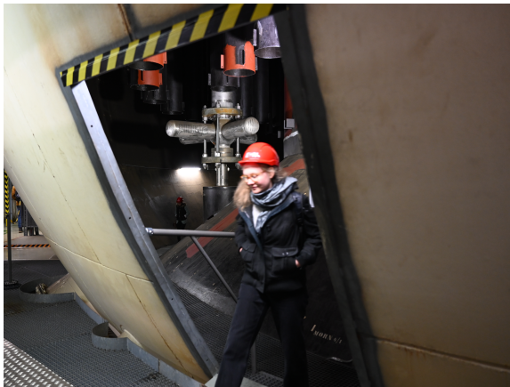
Figure 18: Entrance to the pressure suppression chamber
