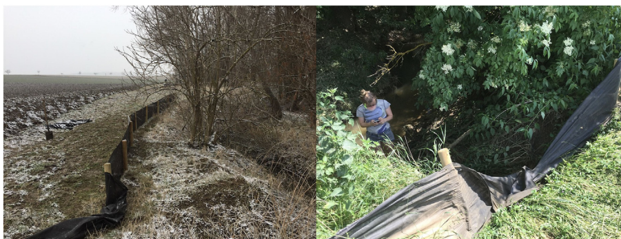
Fig. 5. Riparian buffer strip with sediment fence along a thistle field, where water and sediment retention efficiency investigations have been conducted (see Table 2). Over a length of 150 m, a 1 m high sediment fence made of filter fleece (150 g /m 2 , 100% polyester) was installed at the bottom of a riparian buffer strip (left) in March 2018. Destroyed silt fence at an entry sediment point after a 36 mm/h rainfall event on June 1st 2018 (right). Photos: G. Lützenburg, 2018.
