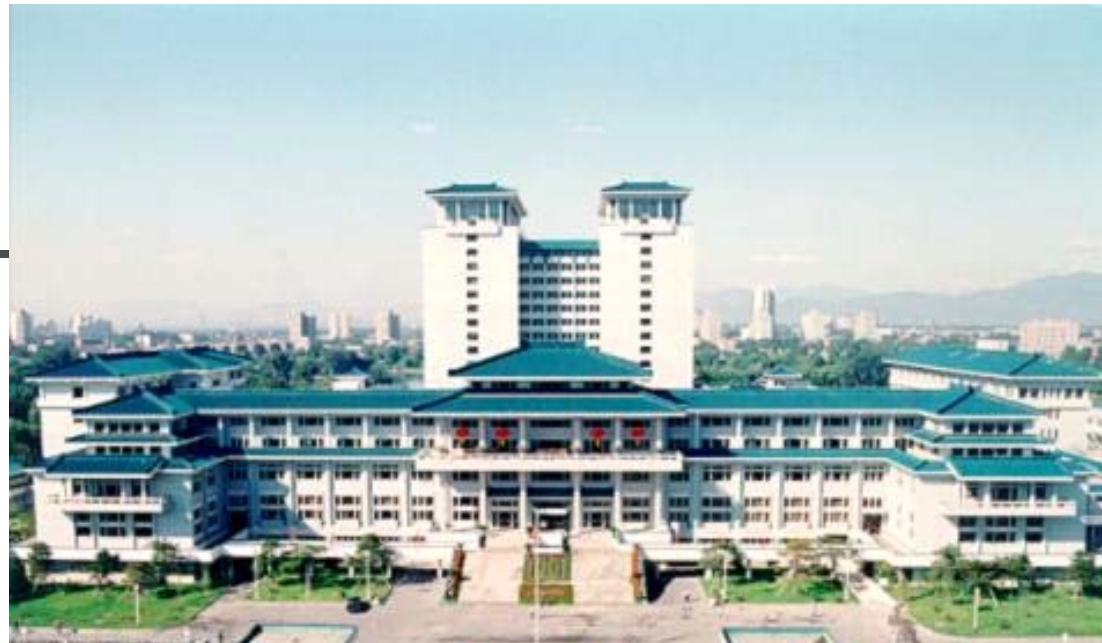
Main building/总馆
